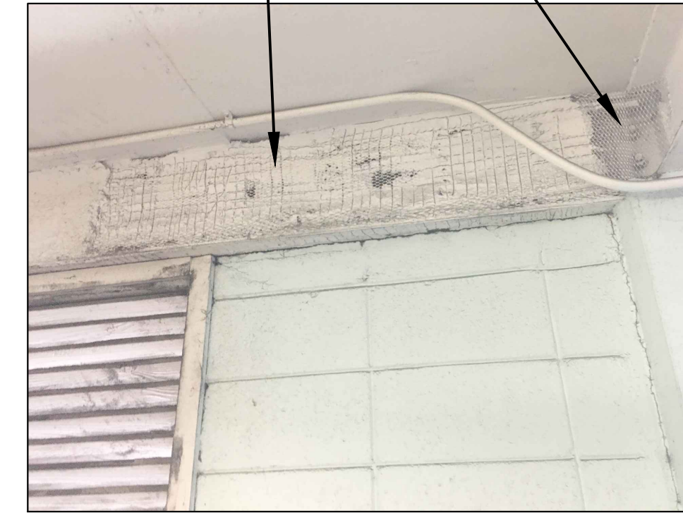
2b) EXISTING METAL LATHE & PLASTER FIRE PROTECTION AT PERIMETER STEEL BEAM. TYPICAL CONDITION. FIELD VERIFY EXTENTS.
