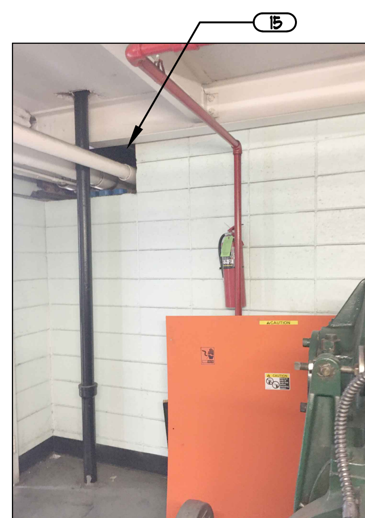
4) EXISTING PENETRATION OPENING TO BE INFILLED.
